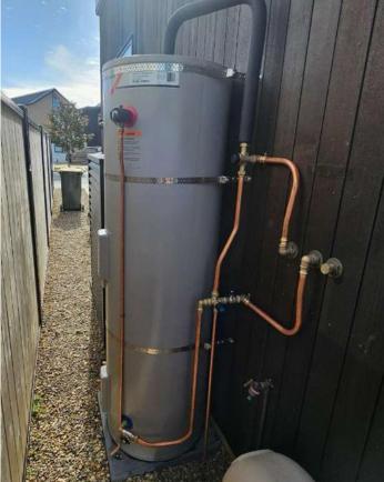
**Please note:** The AquaCore module is not waterproof and therefore requires sheltering from the elements. The homeowners completed this project with a custom heat pump cover.
